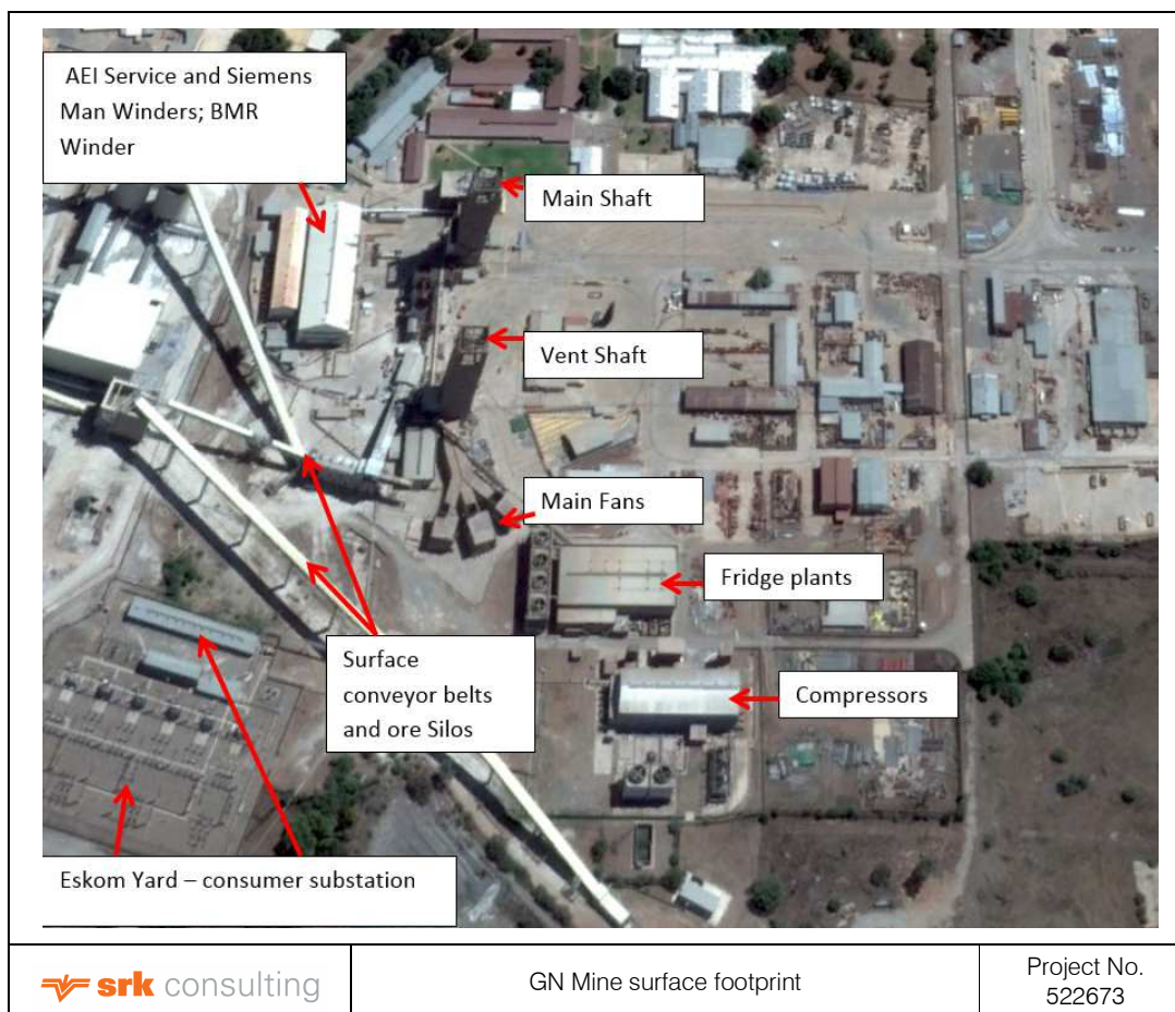
Figure 5.27: GN Mine surface footprint (Source: AngloGold Ashanti)
