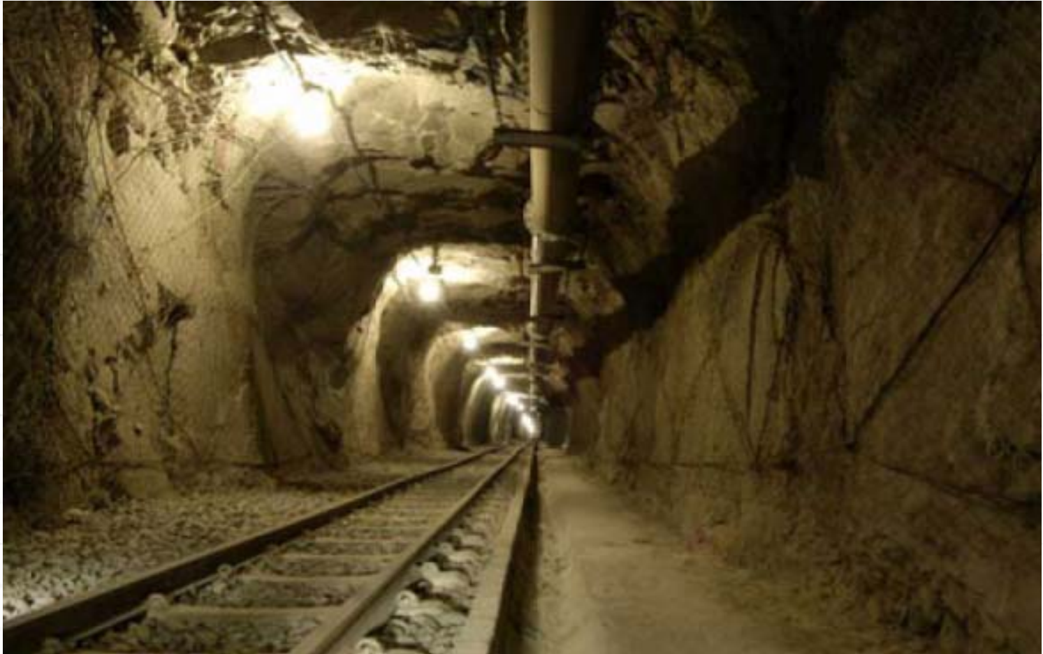
Sub 66 2nd Access Haulage of 1.5 km Equipped with rail line
