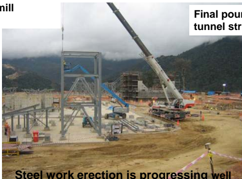
Steel work erection is progressing well
