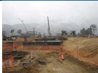
Final pour on main reclaim tunnel structure completed
