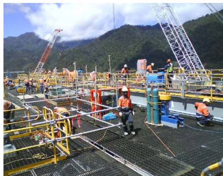
Piping and E&I works on CIL Tank Tops
