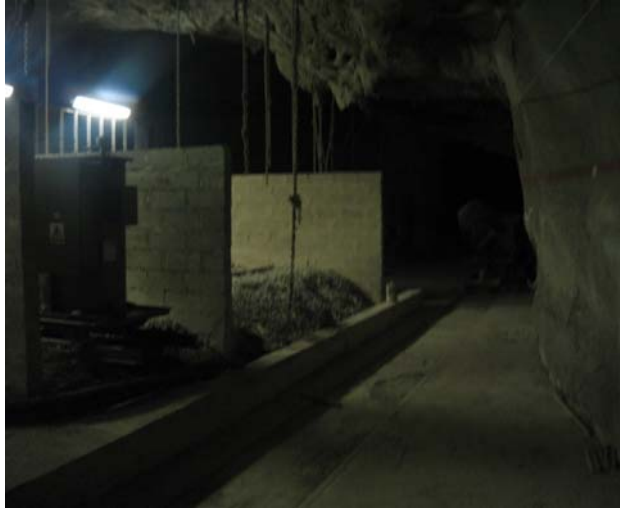
22 kV sub-station under construction
