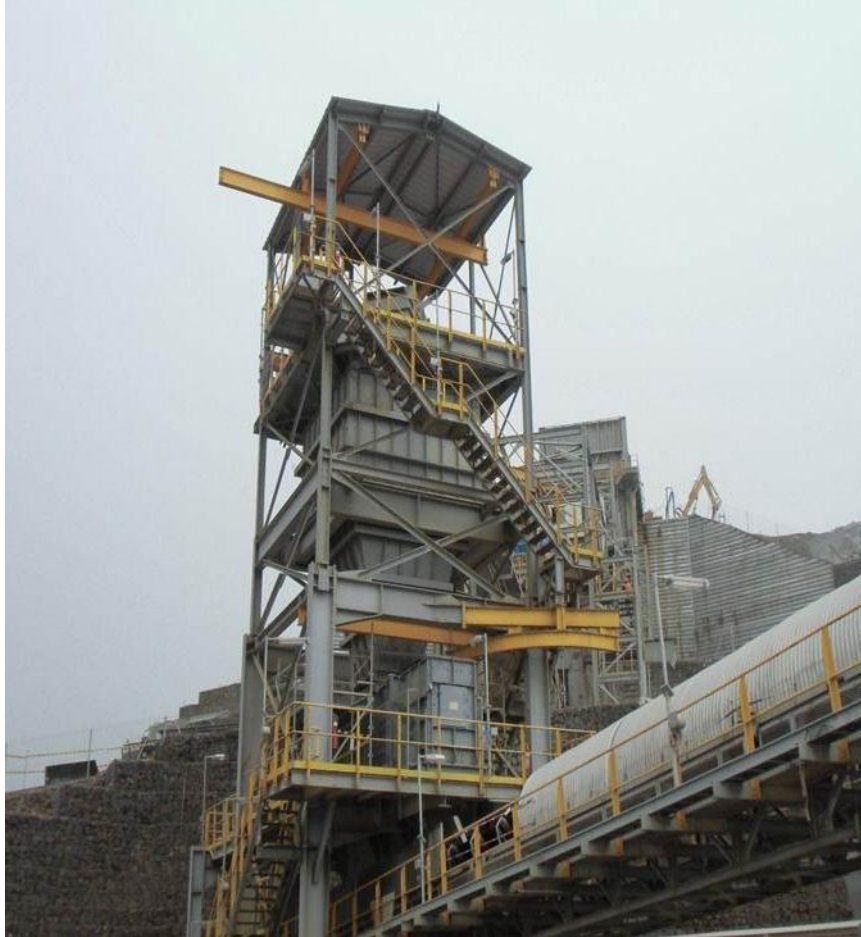
Secondary jaw crusher to be replaced by gyratory cone crusher
