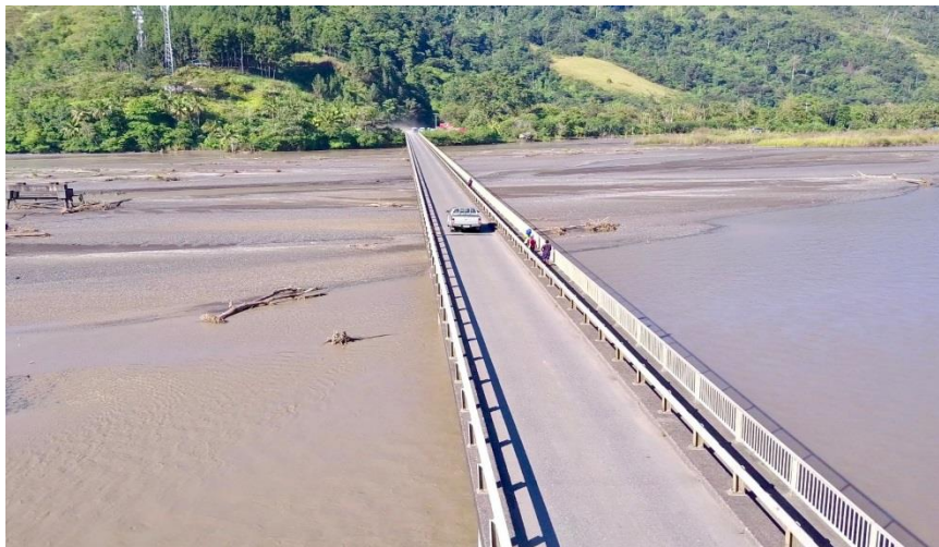
Existing Markham River Bridge near Lae
